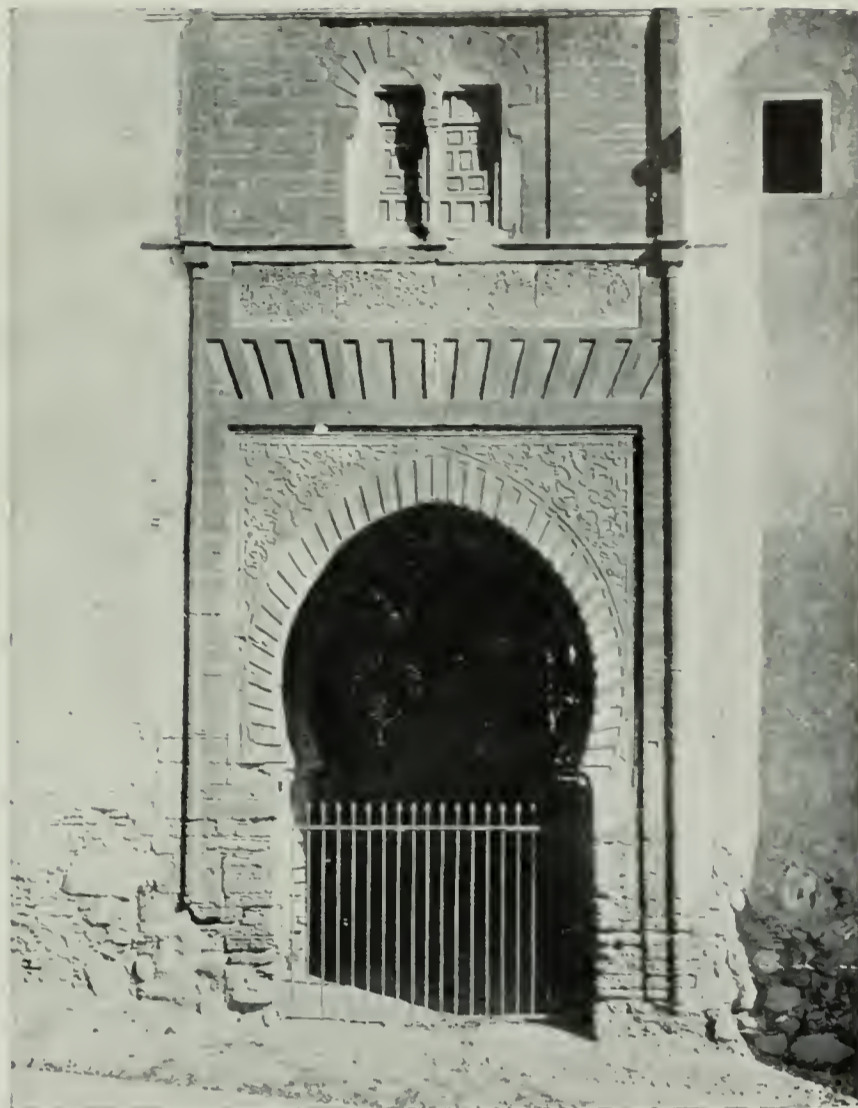
WEST FAÇADE, PUERTA DEL VINO
